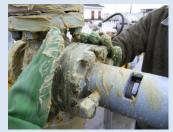
Apply a thin coat Petro-Paste. The Paste shall be applied to threads, cavaties, shoulders, pits and other irregularities.
