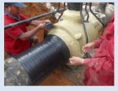
PVC tape recommended for outer protection of Petrol-Tape from mechanical damages and for better isolation from air.
