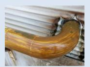
Prepare surfaces by removing all loose scale, rust or other foreign matter in accordance to SSPC SP2 or SP3, After Applying a thin coat of primer to the surface. Then, by hand application, mold the mastic to a rounded configuration to fill irregular shapes or holes and reduce sharp edged surfaces.
