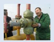
Stuff Mastic in uneven areas such as flanges, valves. Cavaties. The Petro-Mastic shall be molded and packed into irregularities to eliminate bridging and voids.
