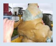
Wrap Petrol-Tape around the surface while applying tension to assure tight tape adhesion.
